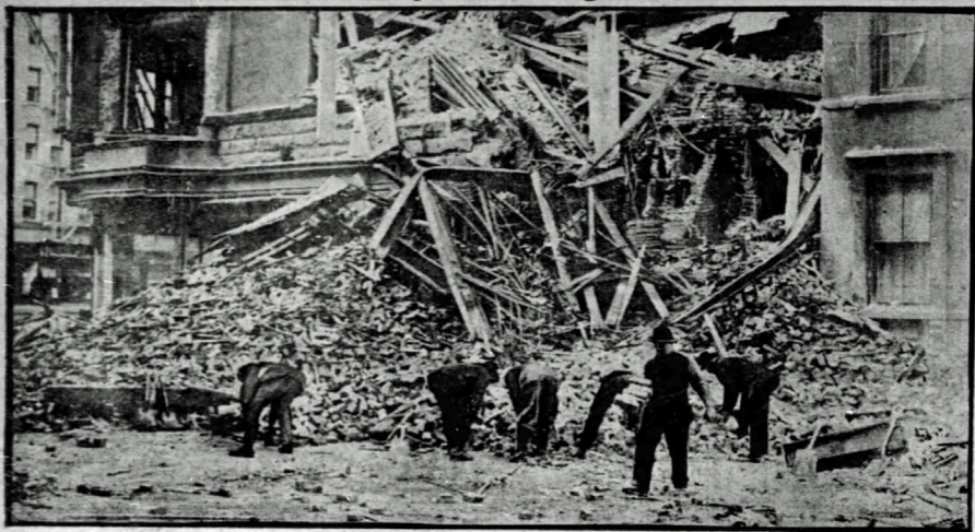
Fifty-Second Street aftermath of Strathmore Apartments collapse in 1920.
